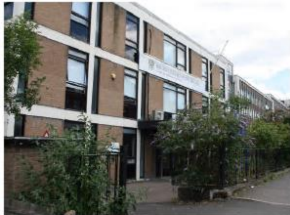
8 | View looking south towards existing main entrance
