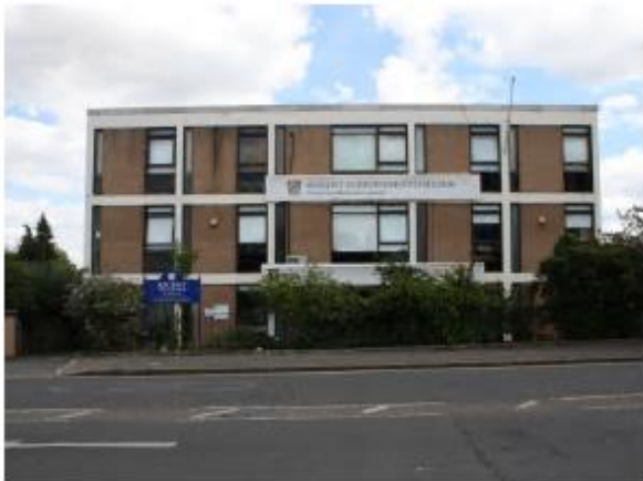
7 | View facing the site from Imperial Drive (looking south-east)
